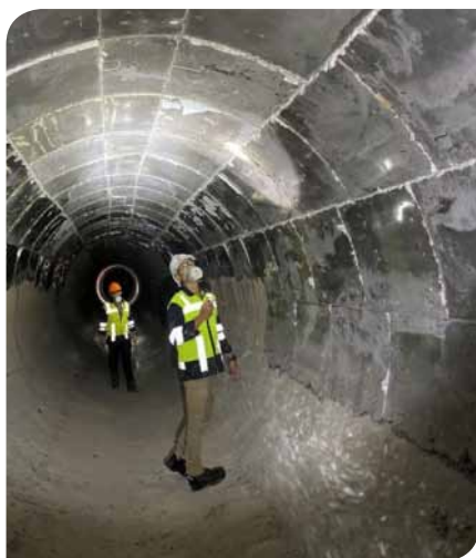
Below: HASLE D59A-ht was used for the tertiary air duct.
