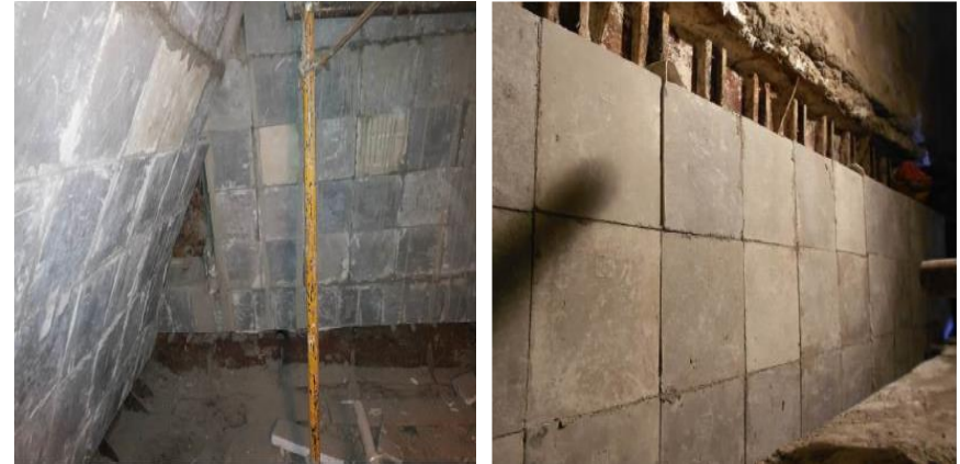
Riser Duct and Smoke Chamber installation
