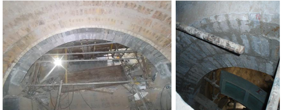
Inlet Arch installation
