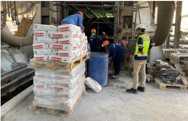
On-site supervision during installation
