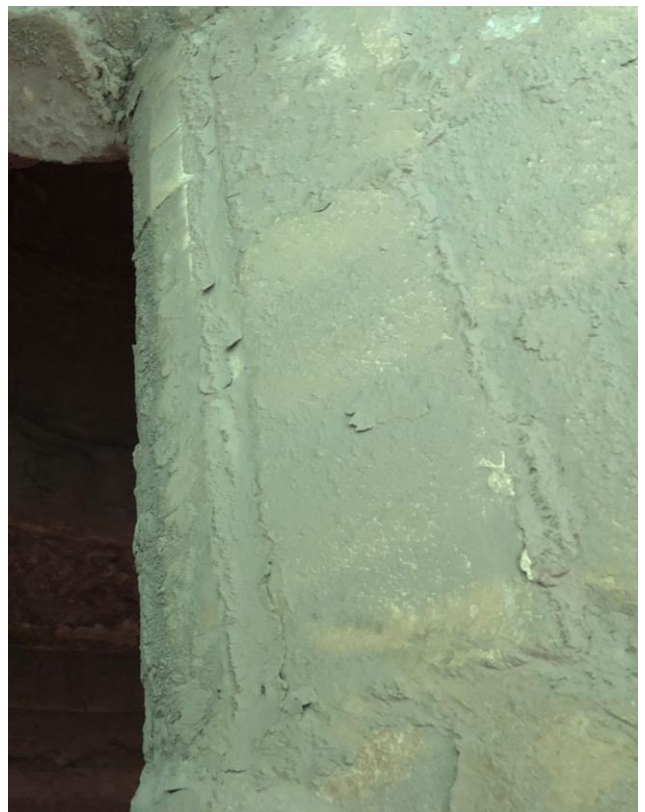
Inspection after 3 years
