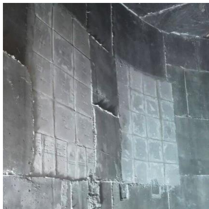
Modular Lining at installation
