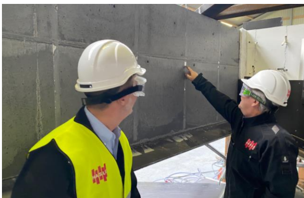
On-site supervision during installation
