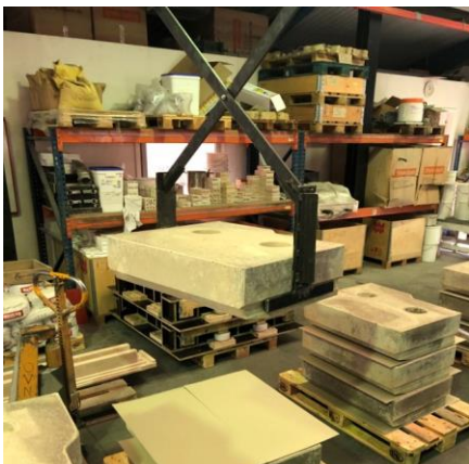
Moving the precast elements by crane
