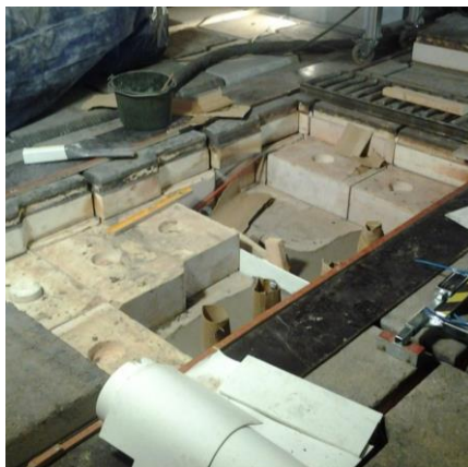
Walking beam furnace under construction
