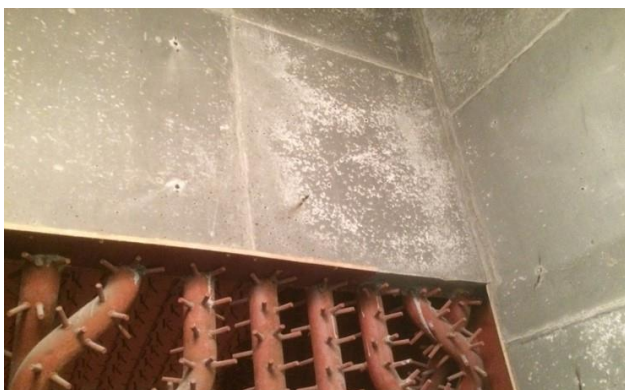
Partly completed wall casting HASLE D39A and D39A-EF
