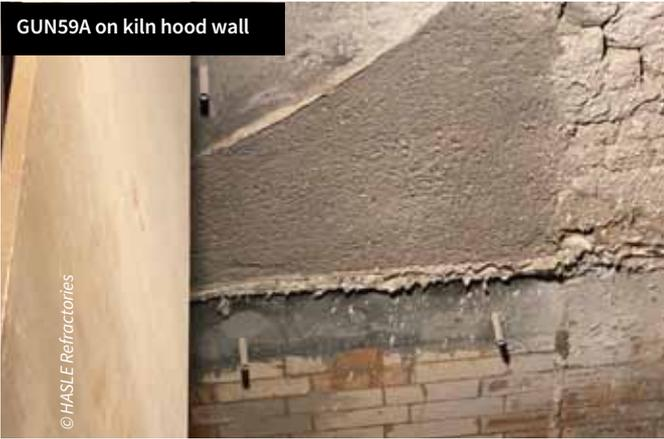
as a precast or in-situ cast solution, it will be good enough for many applications – especially when time is of the essence. Gunning does require a special machine and, most importantly, a skilled operator, for a good result.
