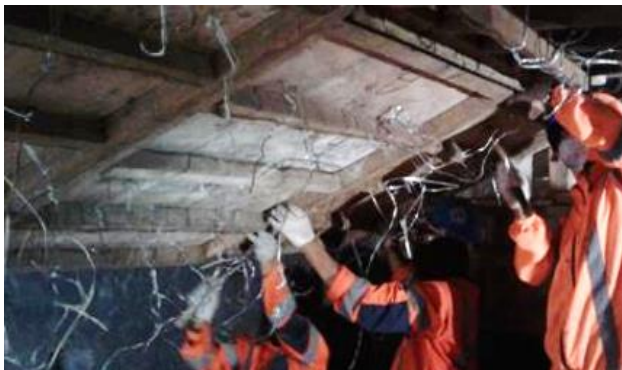
Installing formworks on furnace roof
