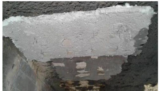
Completed repair using HASLE D59A-ht
