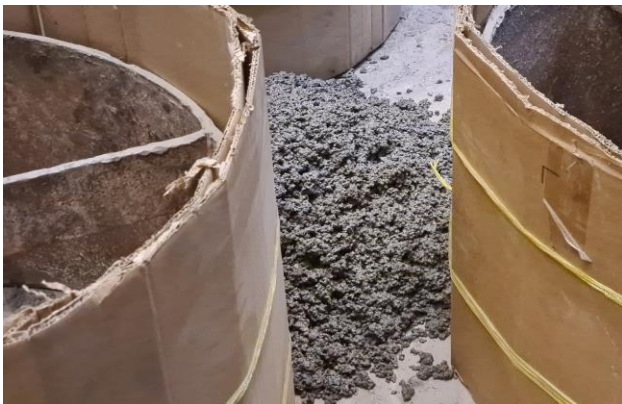
Installation of HASLE D1700A
