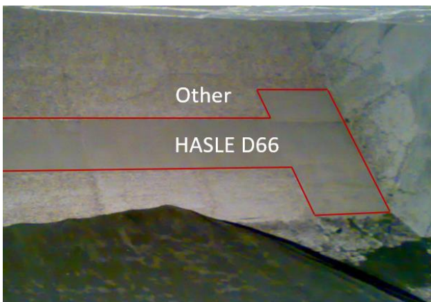
HASLE D66 at installation
