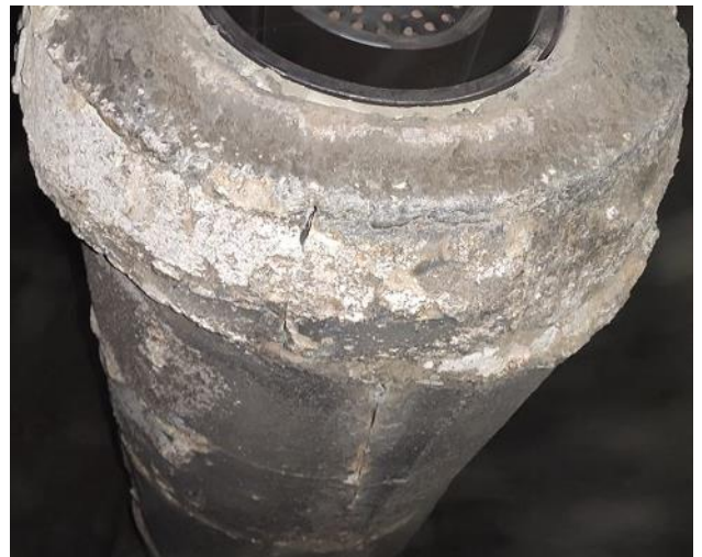
Both images show Burner Pipe with HASLE D52A after 1 year
