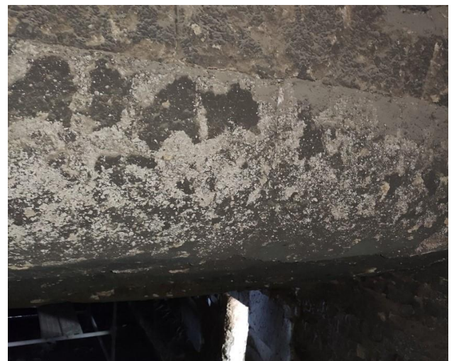
Both images show HASLE D52A on Cooler Bull Nose after 24 months
