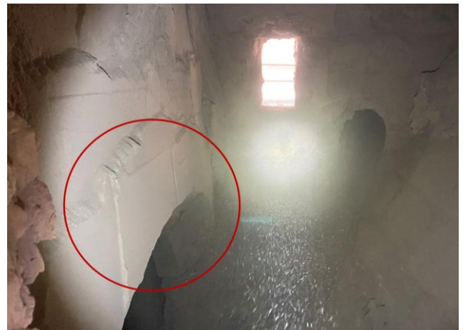
Inspection after 12 months
