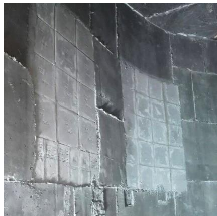
Modular Lining at installation
