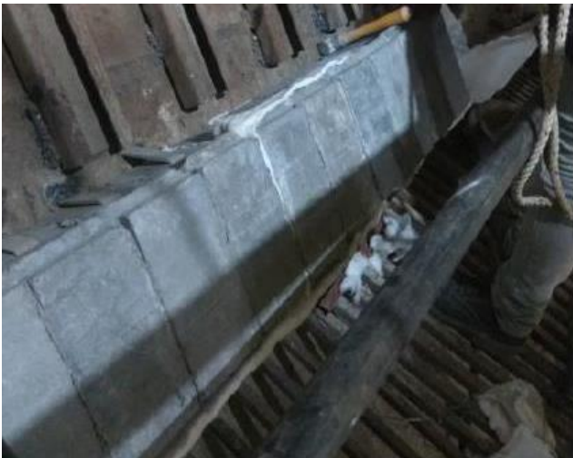
Modular Lining at installation
