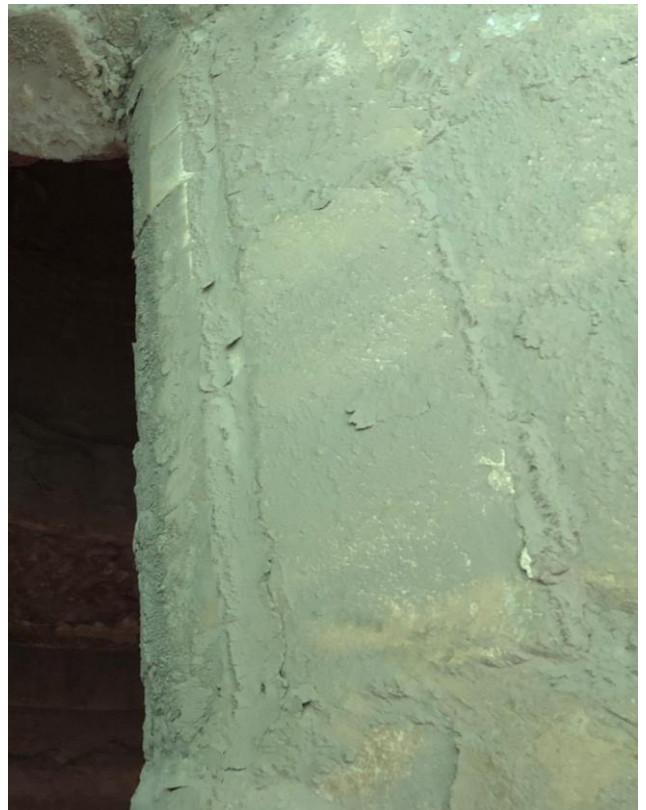
Inspection after 3 years
