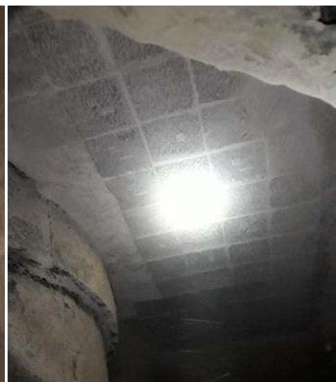
Precast Modular Lining after 3.5 years
