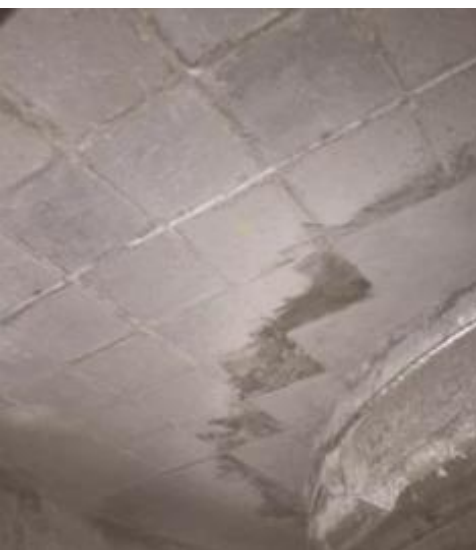
Precast Modular Lining at installation
