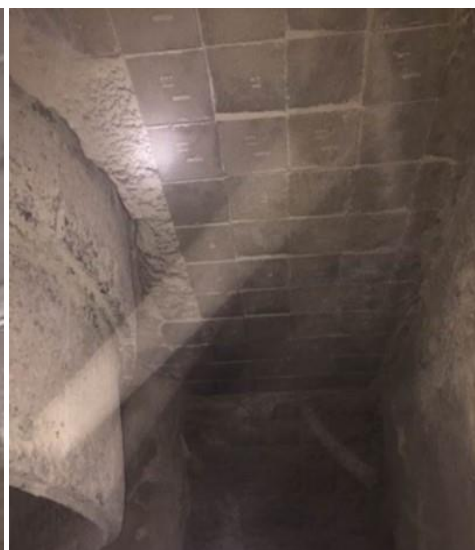
Precast Modular Lining after 2 years
