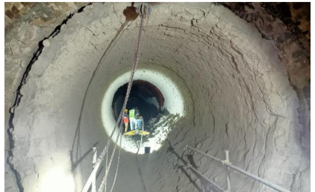
Nose Ring lined with HASLE D52A after 18 months
