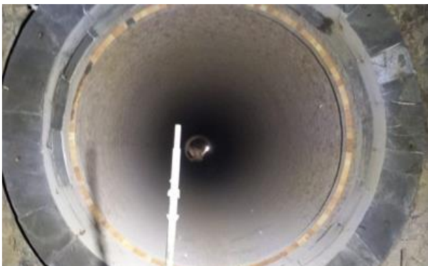
Nose Ring during casting
