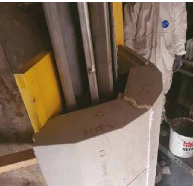
Figure 6: installing the individual HASLE Modular Lining precast elements at W&P Group's Wietersdorf plant in Austria. For maximum flexibility during installation, the elements interlock with a tongue and groove system while the anchors are easily mounted to the wall via a steel rail
