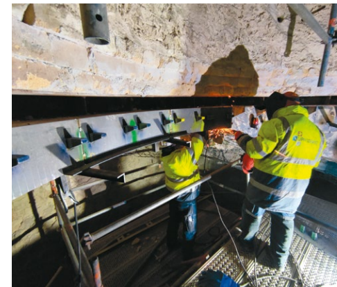
1. A steel support ring is welded to the roof casing of the cyclone.
