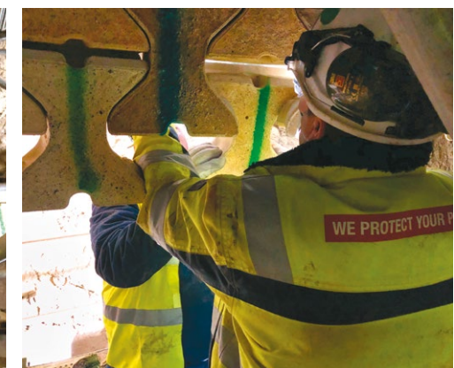
4. Assemble the CVF; The top row of ceramic elements is placed on the brackets on the steel support ring. The remaining elements hang from the elements in the top row.
