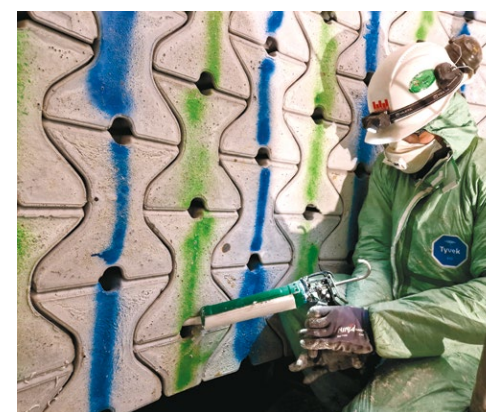
5. The final row of elements is locked in place using a heat-resistant sealant.
