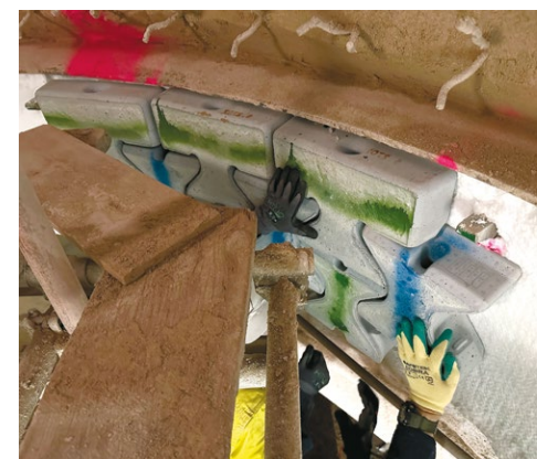
4. Assemble the CVF; The top row of ceramic elements is placed on the brackets on the steel support ring. The remaining elements hang from the elements in the top row.
