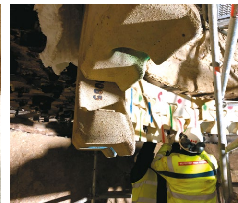
4. Assemble the CVF; The top row of ceramic elements is placed on the brackets on the steel support ring. The remaining elements hang from the elements in the top row.
