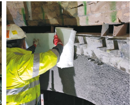
3. Ceramic fiber blankets are placed against the steel support ring to ensure sufficient space for thermal expansion.
