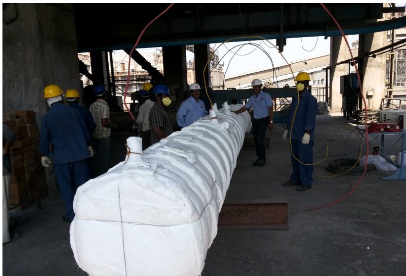
Preheating a burner pipe at Ramco Cements Jayanthipuram Unit, aided by a team of HASLE supervisors.
