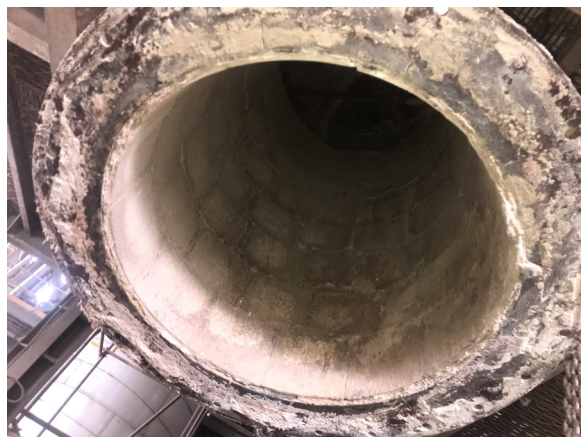
A feed pipe section lined with HASLE precast elements at the cement plant in India after 5 years of operation, with no visible coating.
