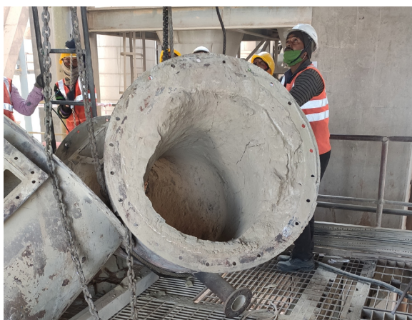
Dismantling feed pipe: heavy coating after one year of operation since last relining.
