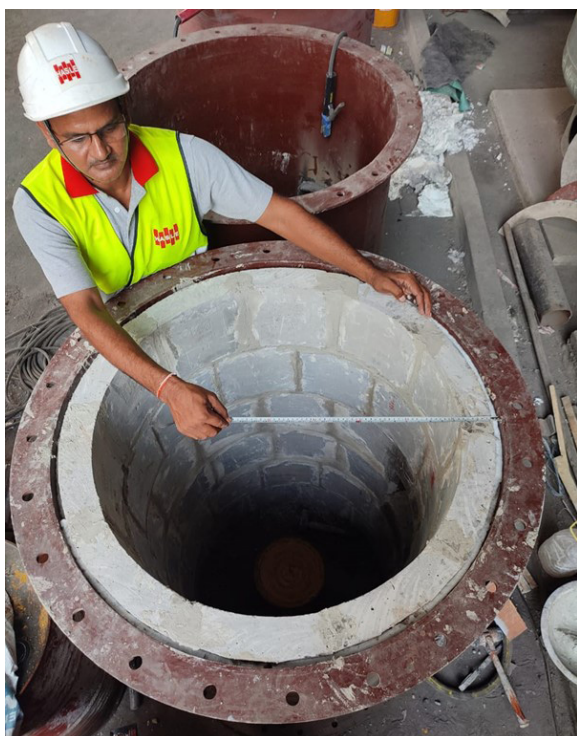
Installation of HASLE cylindrical Modular Lining precast elements in feed pipe sections at a cement plant in India.
