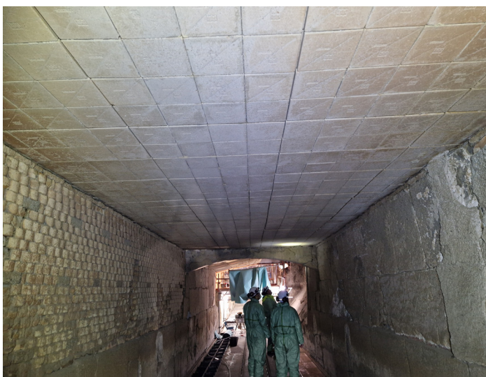
The same HASLE Modular Lining after five years at a German cement plant.
