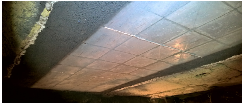
Finished installation of the HASLE Modular lining.
