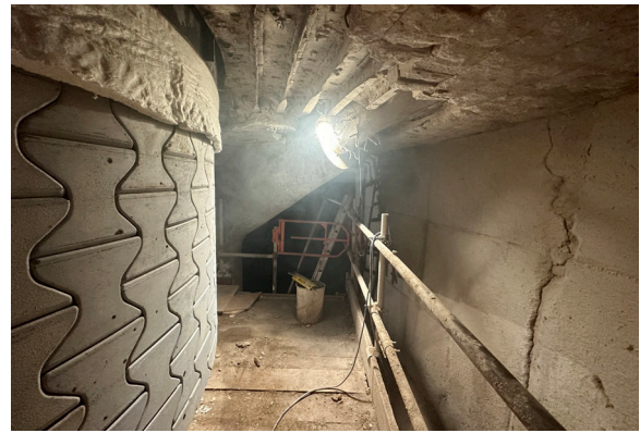
Scaffolding is often required to access the installation area in the cyclone roof.
